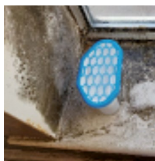
Moisture traps can be purchased from DIY shops and will absorb excess moisture.
