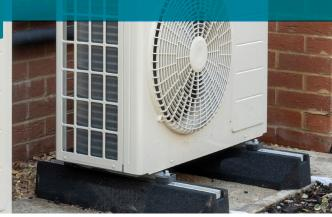
Heat pumps are an efficient and environmentally-friendly alternative to a traditional boiler. Air source heat pumps use the same type of technology as a fridge but work in reverse – they take warmth from outside (even when it's freezing!) and use it to heat your home and hot water.
