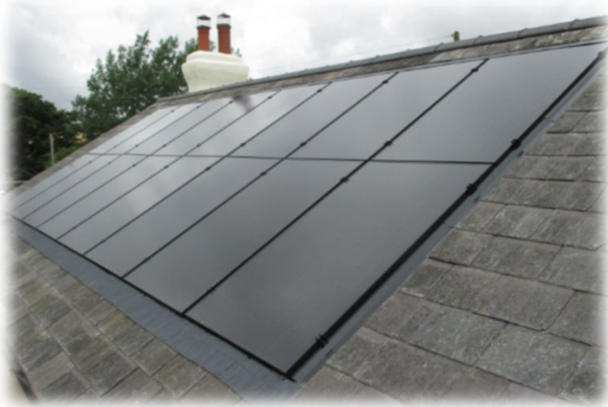
Flush PV Panel Installation
