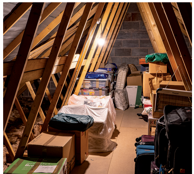
Loft boards and riser kits can be used to create additional storage without damaging insulation.
