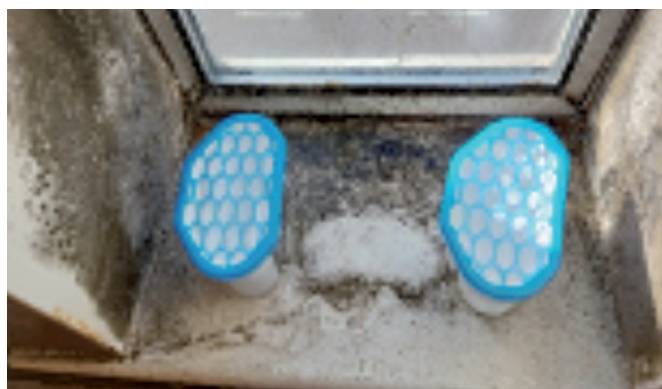
Moisture traps can be purchased from DIY shops and will absorb excess moisture.
