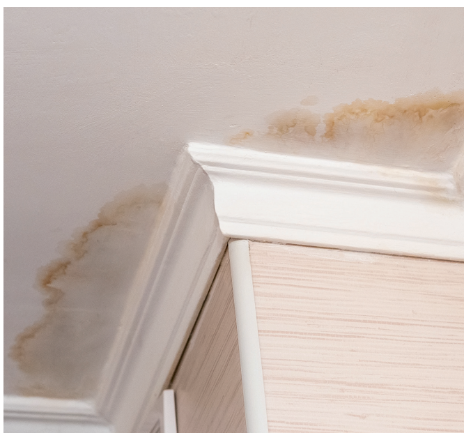
Condensation mould forms on ceilings when moisture laden air condenses on a cold surface.
